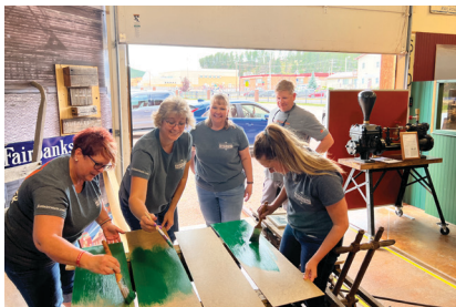
Hill City - SD State Railroad Museum: flagpole installation, model train exhibit, cleanup
