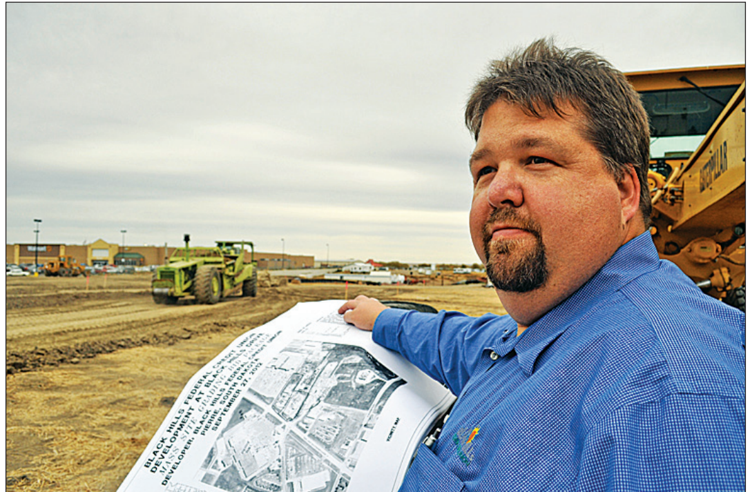
Vice President of Operations Jerry Schmidt looks over the site of Black Hills Federal Credit Union's planned location in Pierre as work begins in October 2012 in this Capital Journal file photo. (Lance Nixon/Capital Journal)
